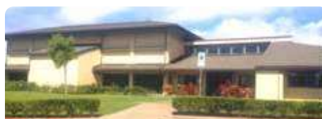
REC CENTER 7 | BUSINESS OFFICE
