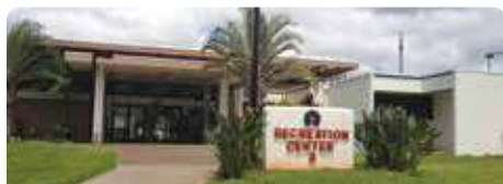
REC CENTER 3 | BUSINESS OFFICE
